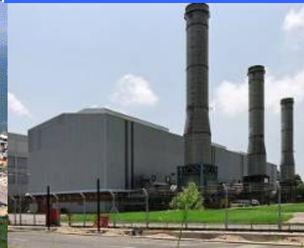
Penny's Bay Power Station
