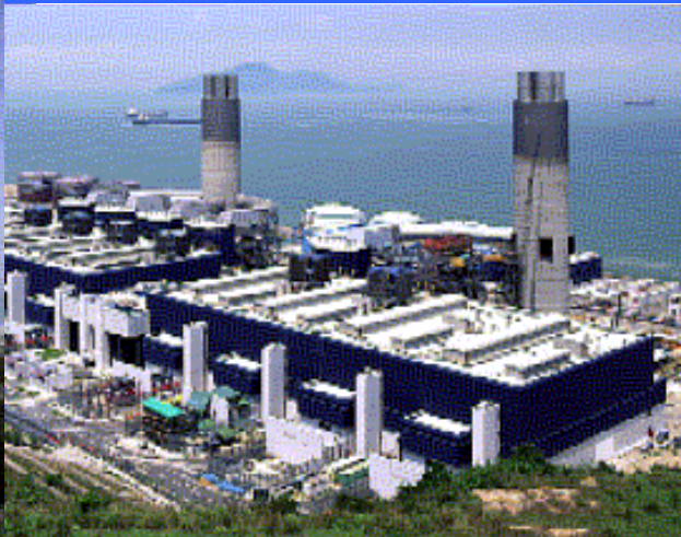
Black Point Power Station
