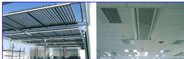
Solar Collector (L) and Active Chilled Beam System (R)
