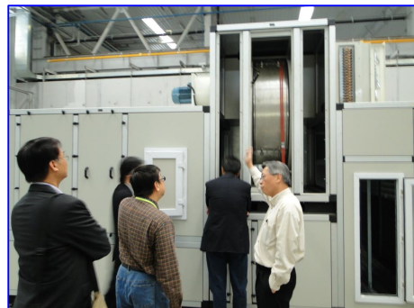
Installation of Desiccant Wheel inside the Air Handling Unit
